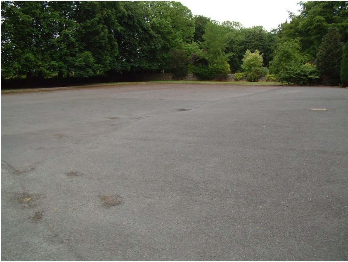
Car Park (Saint Brigid's Church)
