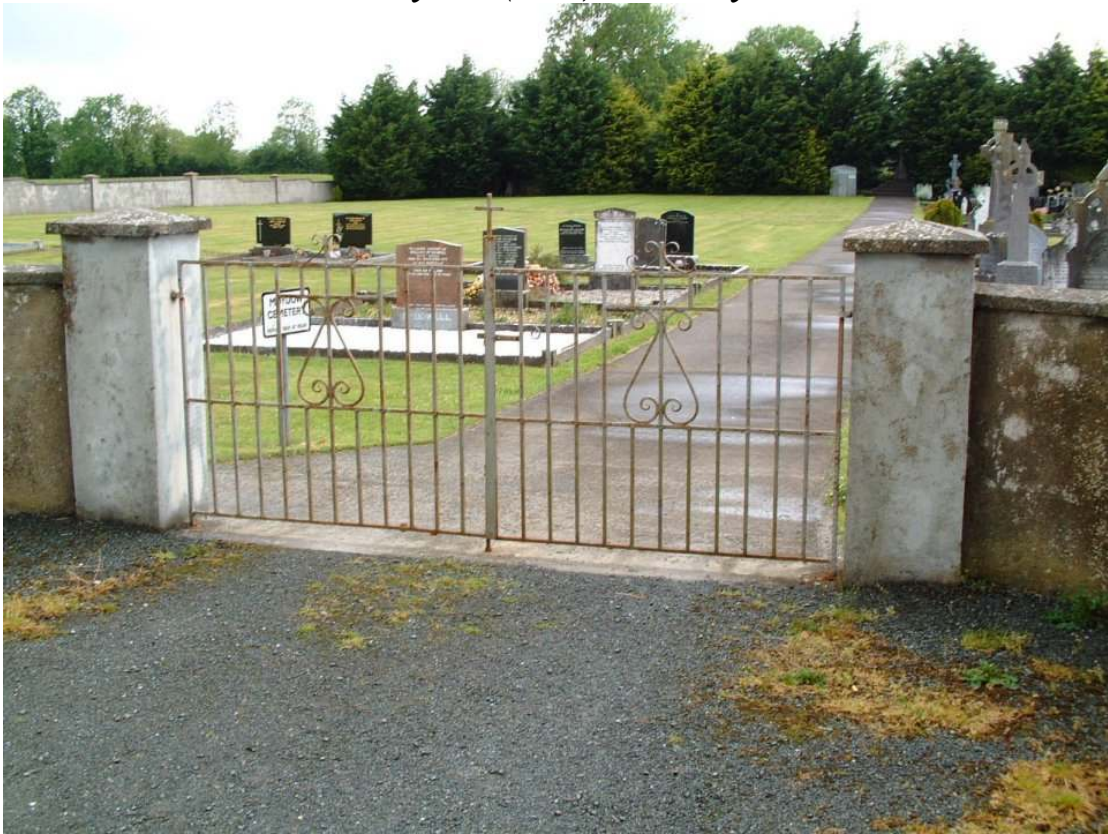
Main Entrance Gate
