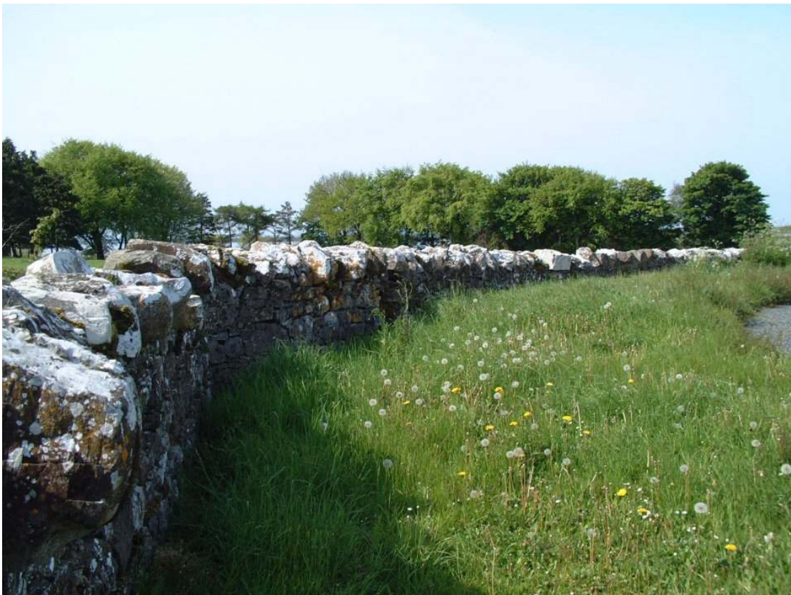
Section of Boundary Wall.
