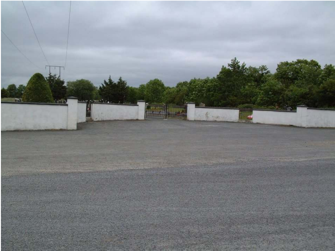
Overview of entrances
