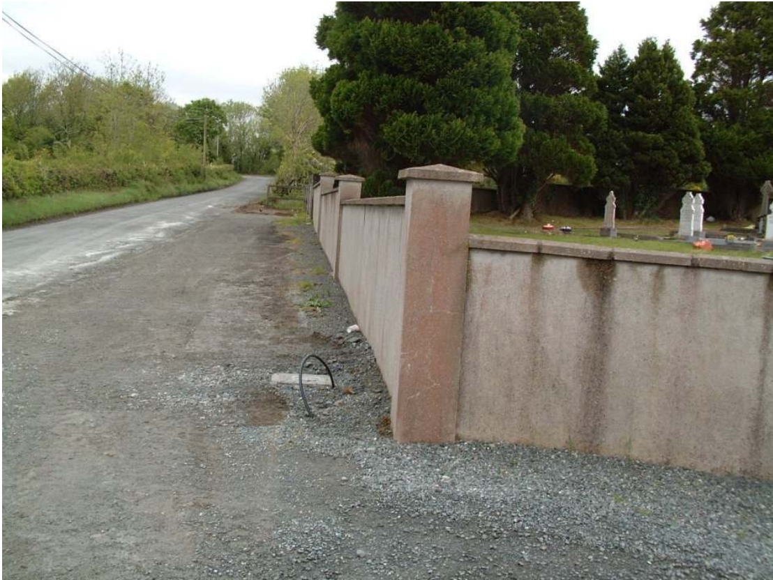
Parking & Part of Boundary
