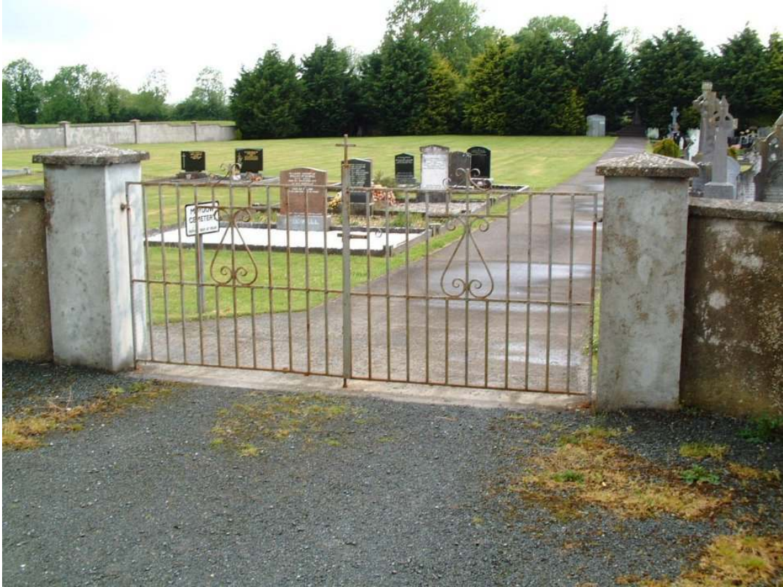
Main Entrance Gate
