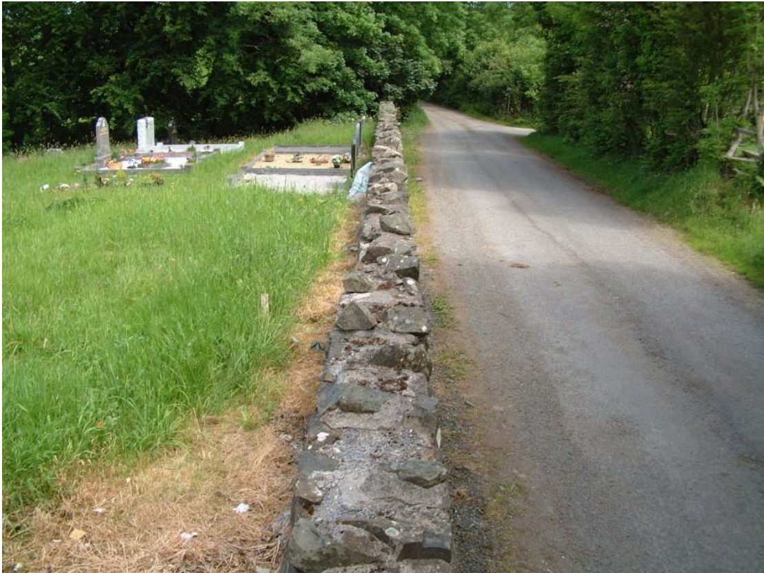
Part of boundary wall.
