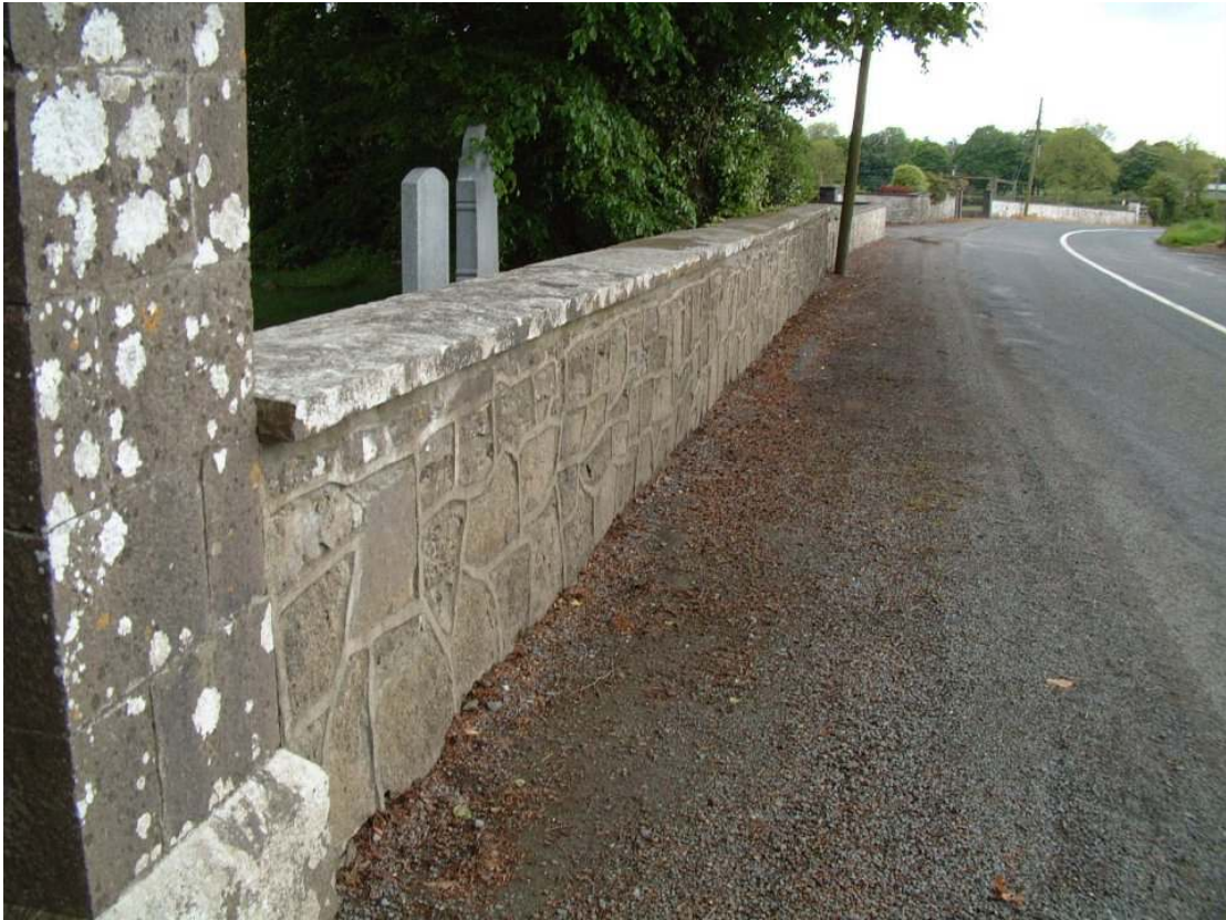
Section of Outer Boundary Wall.
