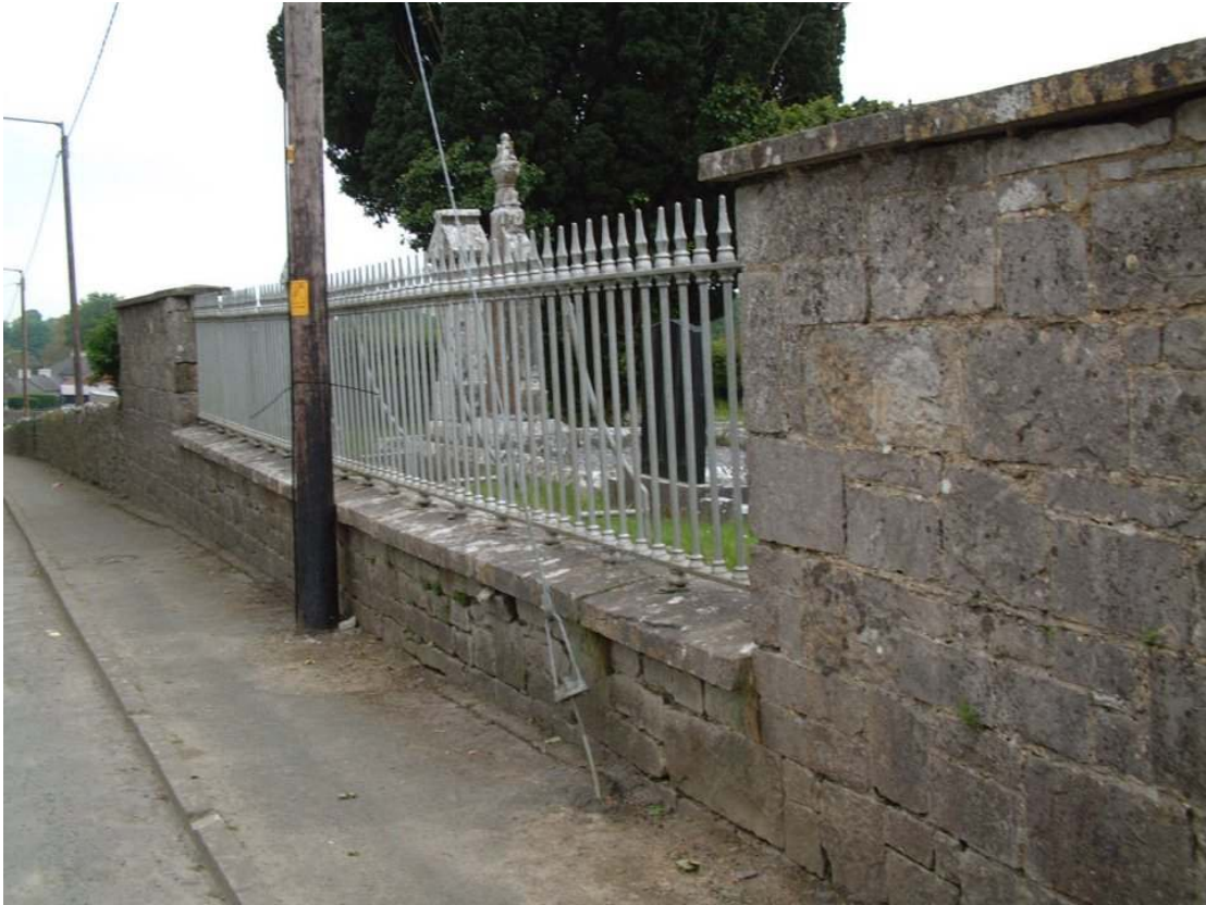
Section of Boundary Wall
